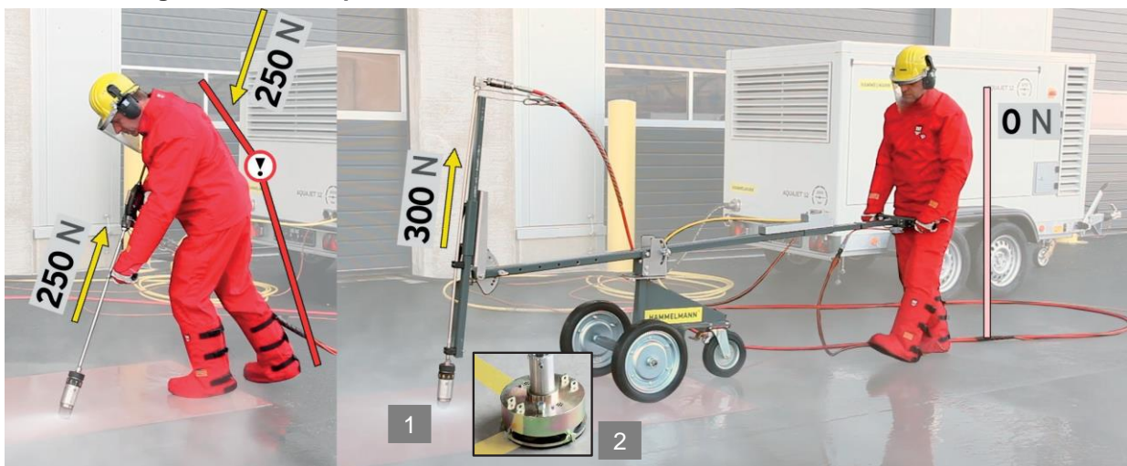
Manual blasting gun work
